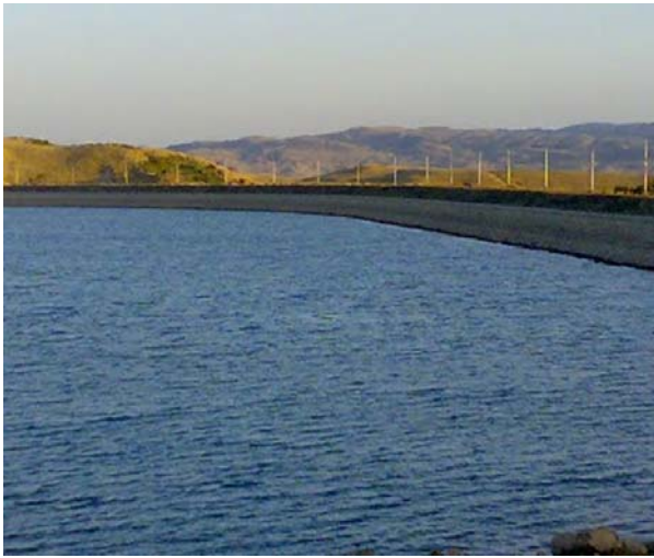
Fig 1: Naryab Dam Overview District Hangu KP, Pakistan.
