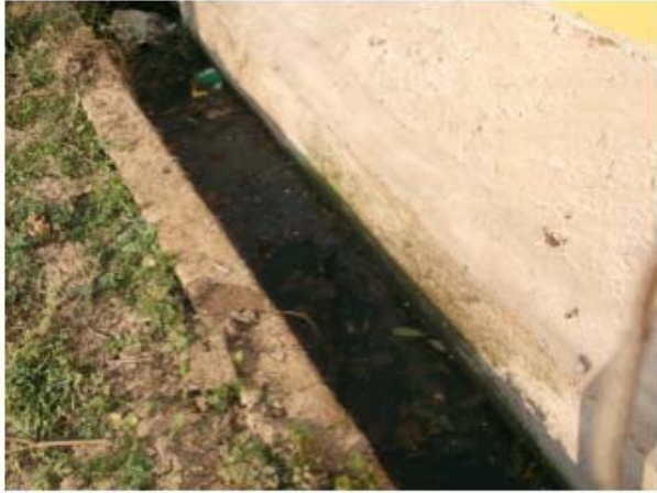
Open type drainage canal
