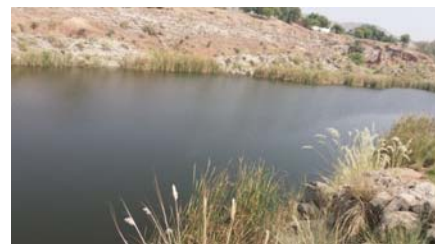
Fig 1: View of Khurram Dam
