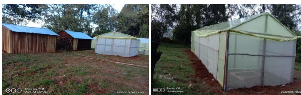
Plate 1(a): Timber walled, mud walled and green house with all flaps open (c) Greenhouse structures L4, L5, L6, L7.
